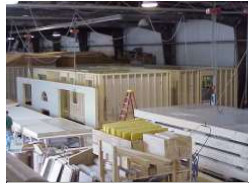
Example of a Dwelling, Manufactured Home Source: http://transportablehomesspecialist.com/
