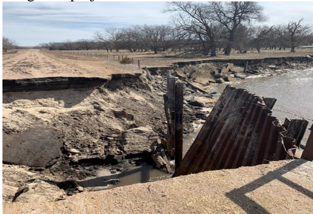
Damage: Loss of east approach and severe damage to wing and abutment. The channel has shifted after making a large bank cut upstream of the bridge. Solution: Possible channel stabilization, Possible remove and replace wing and abutment, Possible new structure. Status: We will develop repair plans and estimates for FEMA to determine if structure would qualify for replacement or mitigation. Visit with NRCS to determine if they would participate in bank stabilization. Cost estimate: $800,000 County share would be split with Knox County.
